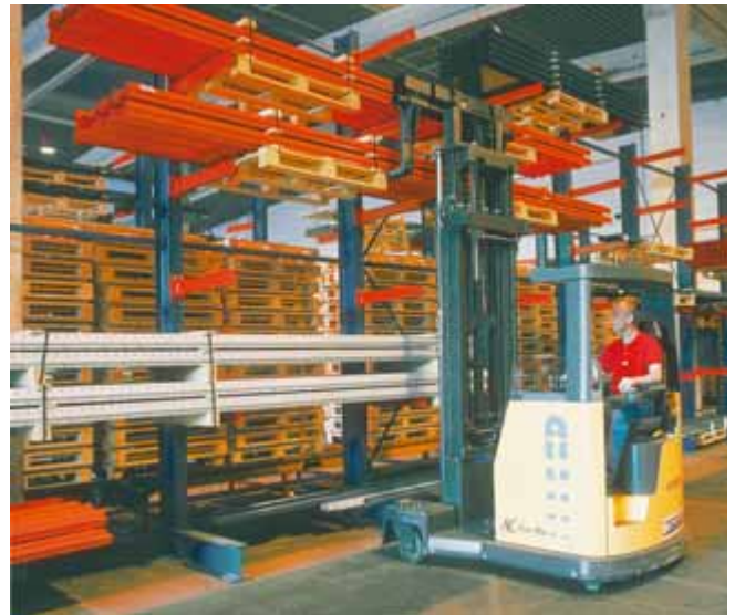
Flexible handling in cantilever racking for handling at higher levels the driver leans back and the seat tilts 15 degrees..
